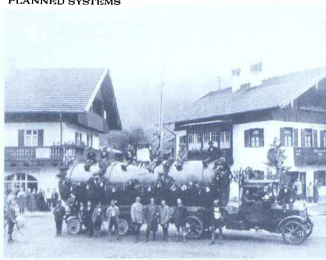
Figure XII.9. Transporting a section of penstock to the Walchenseer power plant, 5 May 1924. Courtesy of the Deutsches Museum, Munich.
