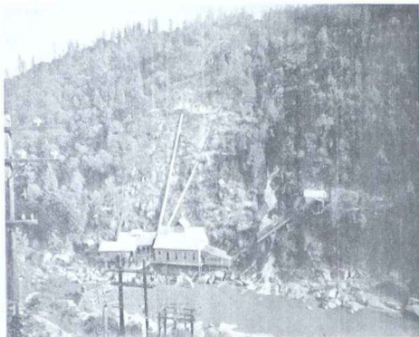
Figure X.5. Nevada power plant: Low-head and high-head penstocks (rear). Courtesy of the Pacific Gas & Electric Co., San Francisco, Calif.
