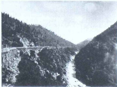
Figure X.7. Flume line to Colgate power house. Courtesy of the Pacific Gas & Electric Co., San Francisco, Calif.
