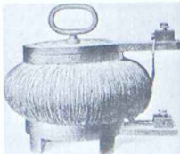
Figure IV.7. The Déri, Bláthy, and Zipernowski transformer, 1885. From Fleming, The Alternating Current Transformer . 2: 87.
