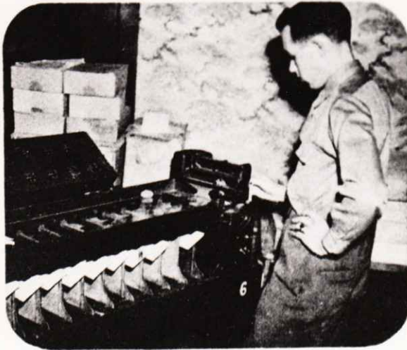
10. HOLES ENABLE CARDS TO BE ELECTRICALLY SORTED AND TABULATED; 7 PER SECOND
