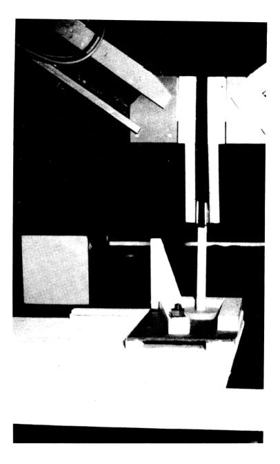
Fig. 13.2—FREDDY uses a crude vice to clamp a wheel while fitting in the axle. The car body and another wheel can be seen in the background.
