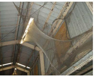
Fig. 12. Hanging 8' light fixture (2.44 m long) pulled out of alignment by webbing.
