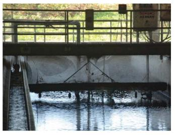
Fig. 8. Webbing beneath traveling bridge.
