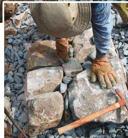
There will be voids. Face stones don't have to meet tightly inside the wall. Just pack the spaces full of hearting stones.
