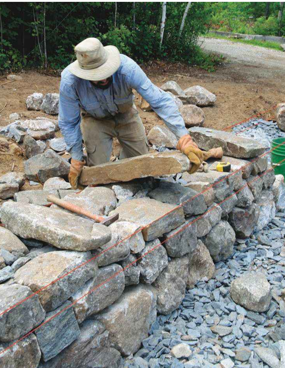
Tie the sides together. It's typical to let through-stones extend 1½ in. past the wall face to allow for flexibility in their length and for the wall to settle without slipping off them.
