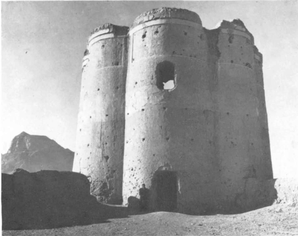
Pl. I. The west tower in the Hazār Jarīb, 1963. See plan in Fig. 2. Believed to be built c. 1700
