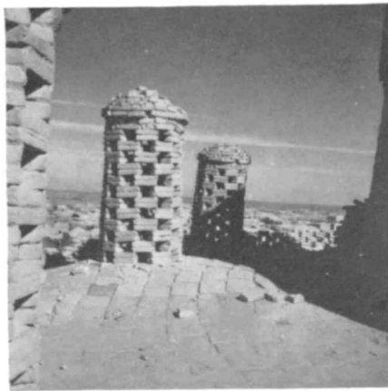
A tower immediately north of Isfahān Pl. IX. Turrets through which pigeons enter the tower
