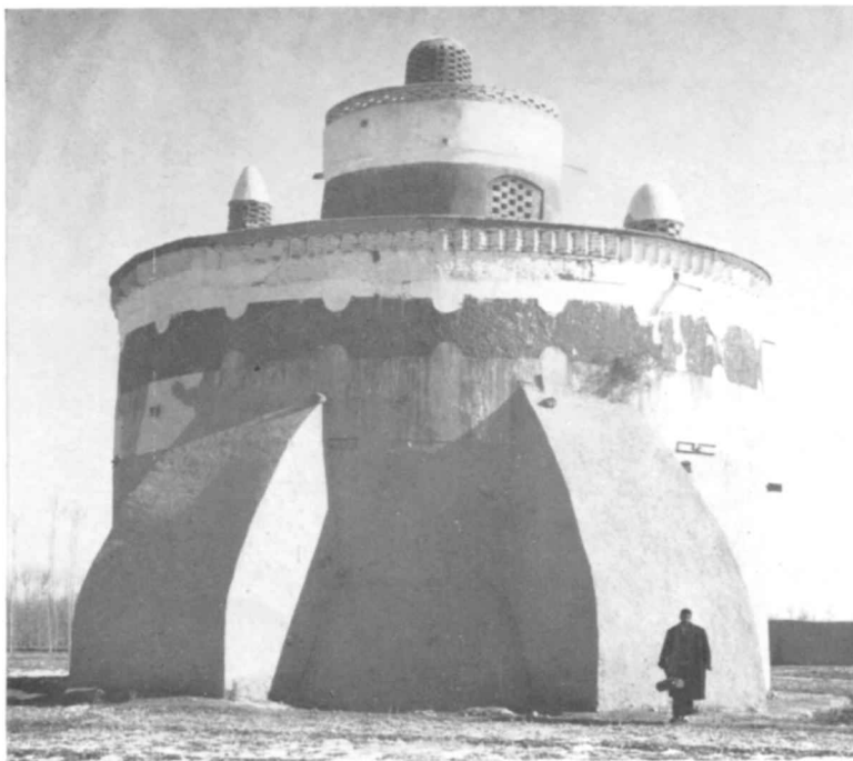
Pl. XI. Smooth plaster bands were to prevent snakes climbing the towers, but their function seems to be undermined by the addition of buttresses. A tower near the Ateshgāh
