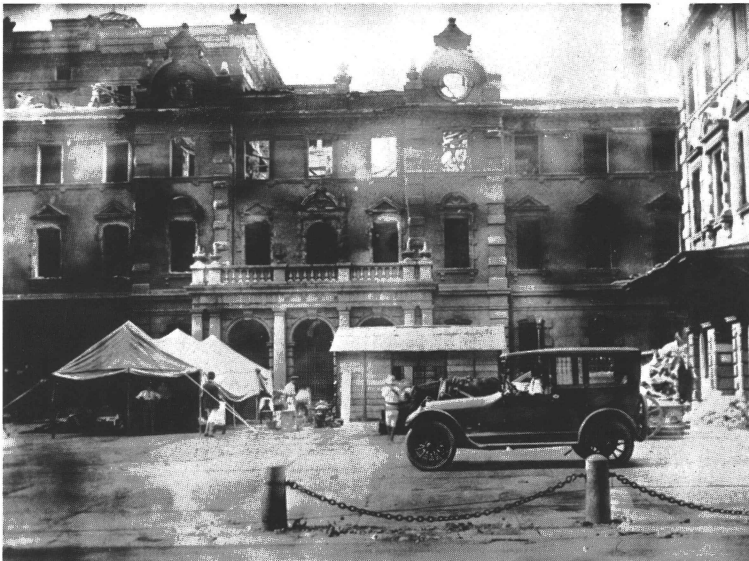
24. Mitsui Gomei building in Tokyo, after the Great Kanto Earthquake of September 1, 1923.
