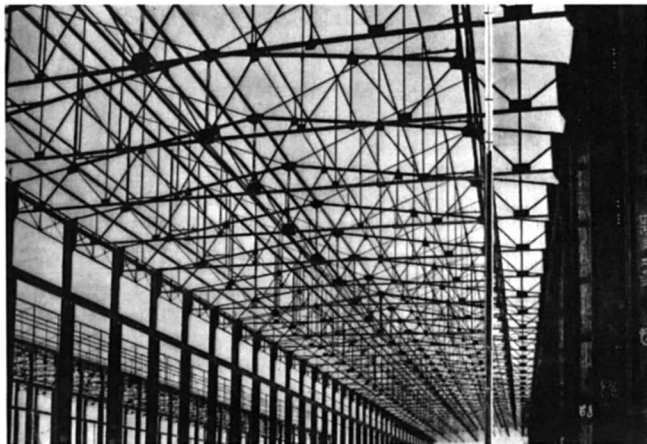
Figure 10. Construction of assembly shop at Nizhnii Novgorod (Gorky) Automobile Plant. USSR in Construction , no. 3 (1933).
