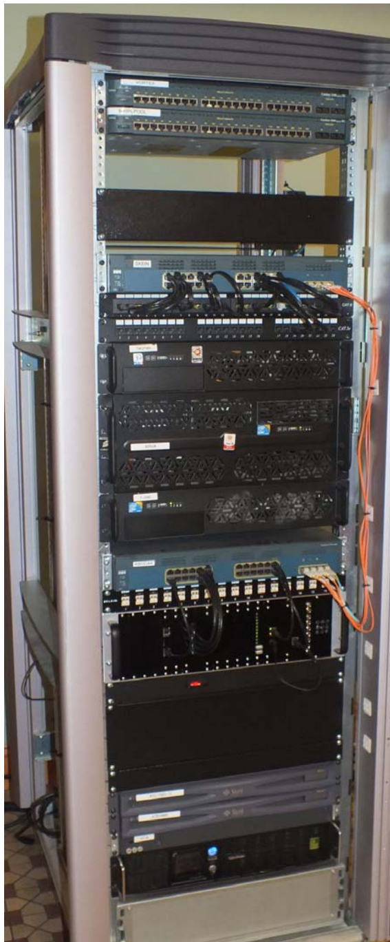
Figure 4.6: FPGA cluster on rack
