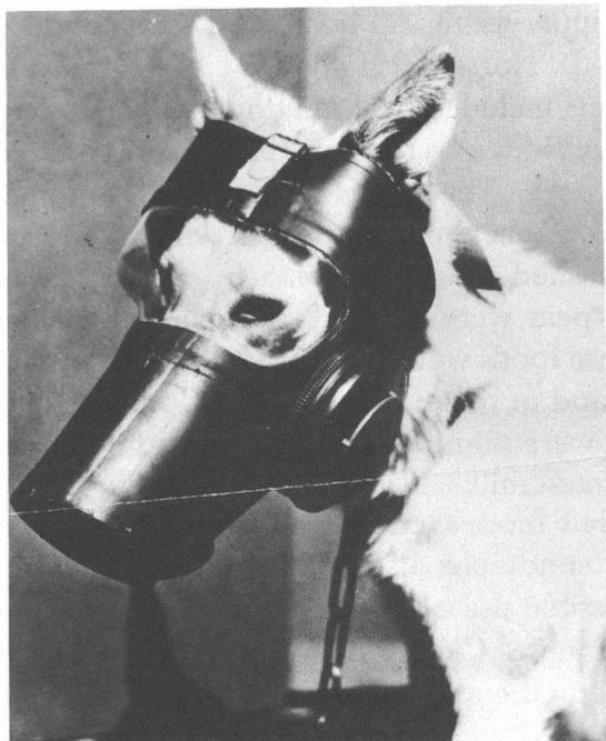
Lassie gets fitted with a gas mask. The M6-12-8 mask weighed slightly over two pounds and could fit about 97 percent of the dogs in service. (*Carlisle Barracks*)
