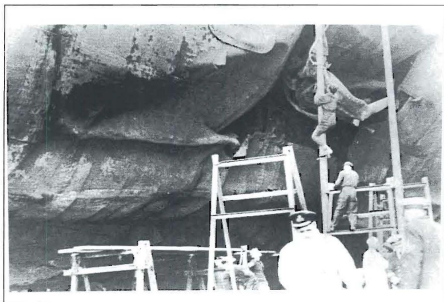
Figure 3-7. Damage Sustained by the HMS VALIANT. (Imperial War Museum)
