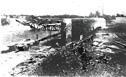
Figure 2-23. The Bridge at Canne Hours After Being Destroyed by the Belgians.
