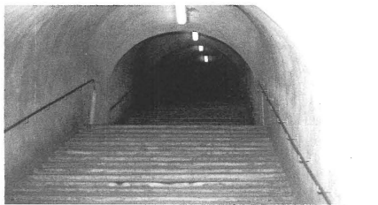
Figure 2-8. Tunnel Leading From Upto Second Level. (Author's Photo)
