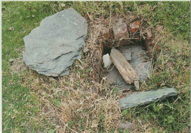
A sump hole built by Bakewell for his irrigation works at Dishley.
