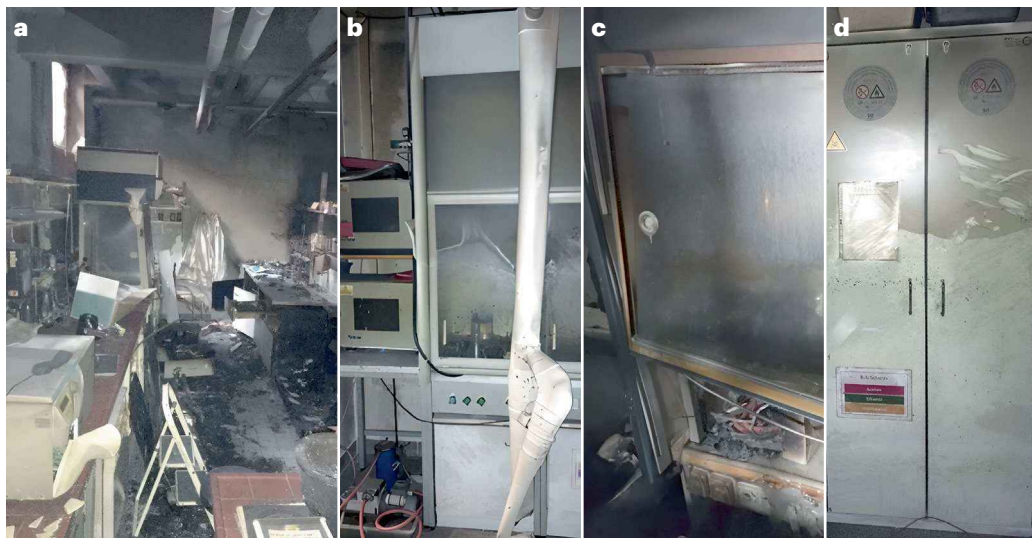
Fig. 2 | Photographs taken after the fire. a–d, Burnt-out laboratory K05 (a), collapsed air extraction system (b), destroyed fume cabinet (c) and the level of the firefighting foam indicated against a chemical cabinet (d). Credit: Christian Tisch.
