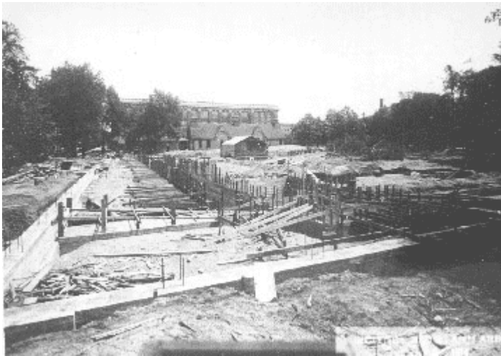
The construction of the Natural Science Building, 1914.
