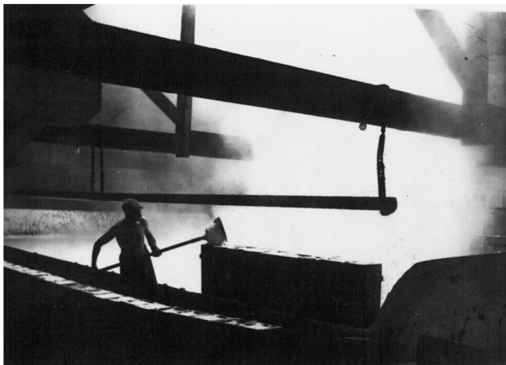
Fig. 1. Filling wet salt into a tub. Middlewich c. 1960.
