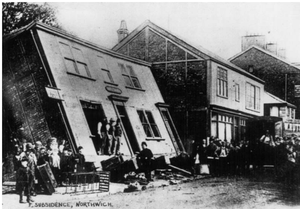
Fig. 3. Subsidence, Northwich c. 1900.
