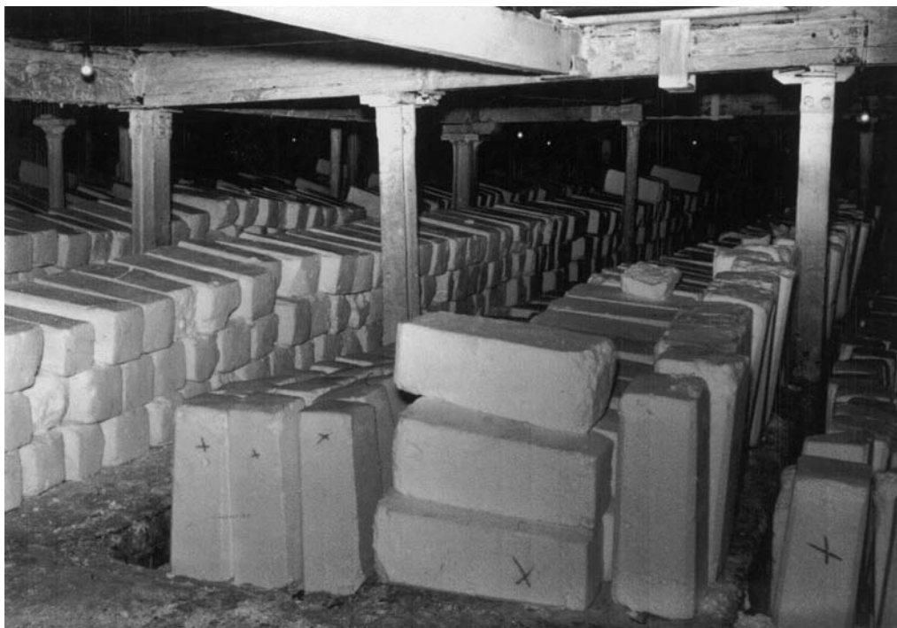
Fig. 2. Lumps drying in hothouse. Middlewich c. 1960.
